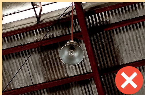
Image 24. Lighting fixtures without enclosure
