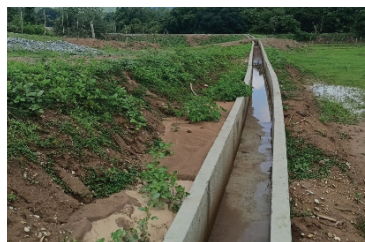
Construction of San Aurelio SWIP 1st Canal Lining in Brgy. San Aurelio, Balungao, Pangasinan
