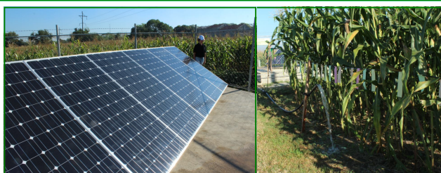
Left photo is the solar irrigation system established in INPC Batac, Ilocos Norte, used to irrigate corn during summer.
