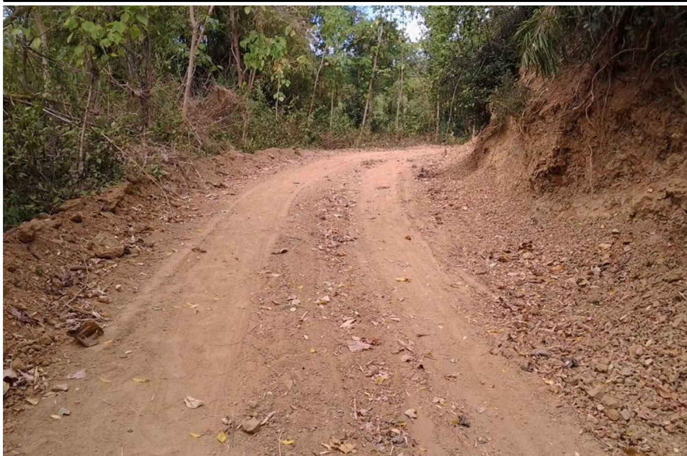
Proposed I-BUILD sub-projects of Ilocos Sur—the Rehabilitation of Tubigay-Baracbac-Nagcullooban FMR in the municipality of Sinait
